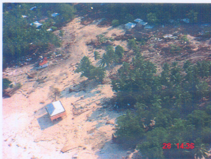
An aerial photograph of the damages caused to houses by tsunami
