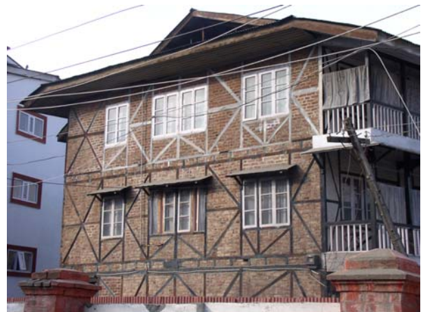
Photo.12:- Srinagar – Good example of Dhajji type of wall.
