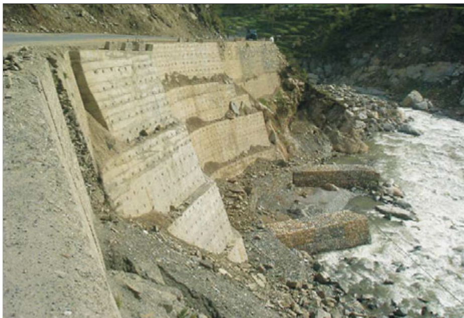
Figure 7.9: Transverse spurs along river sides to reduce toe erosion
