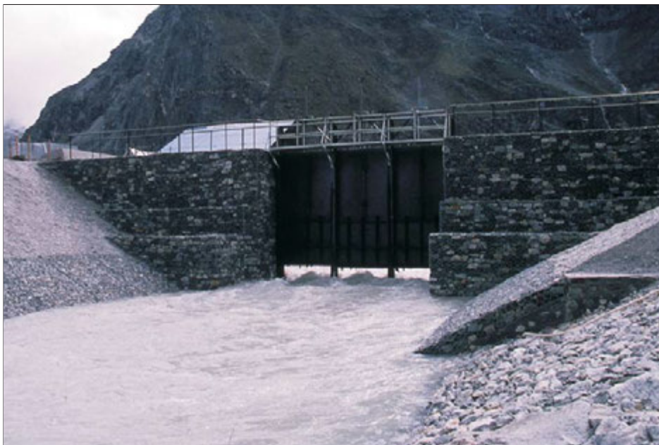
Figure 7.12: Channel for creating outlet form glacial lakes
