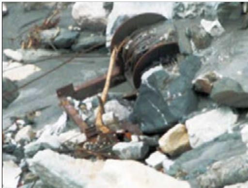
Fig.4.59: Equipments of the Power Project were damaged and washed away by flashfloods
