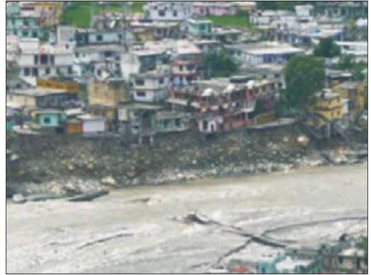
Fig.4.28: Eroded river bank put buildings at risk after the flashfloods in Bhagirathi river
