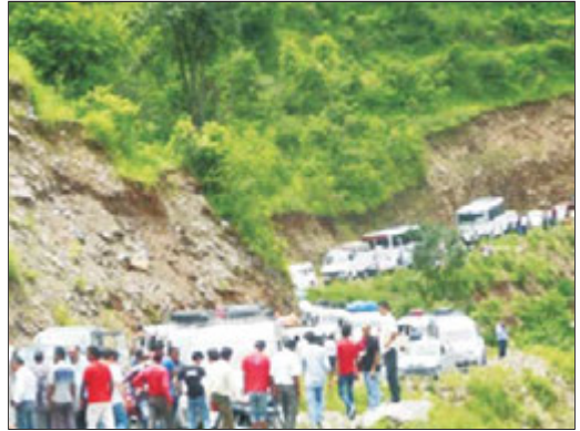
Fig.5.32: Road traffic disrupted due to landslides on way to Uttarkashi
