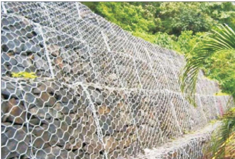
Figure 7.4: Gabion wall made with wire crated boulders used for landslide mitigation
