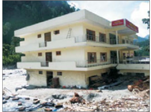
Fig.4.4: A panoramic view of the damaged hotel building situated near Asi Ganga River at Gangori
