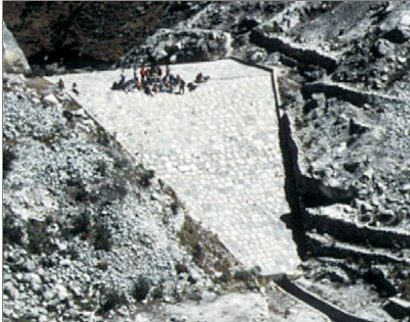
Figure 7.13: Channel and moraine dam built in reducing impact of GLOFs.
