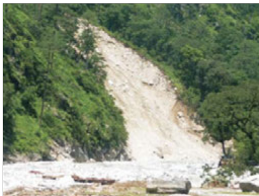
Fig.4.43: Landslide due to toe failure near river bank after flashfloods in Asi Ganga River at Gangori
