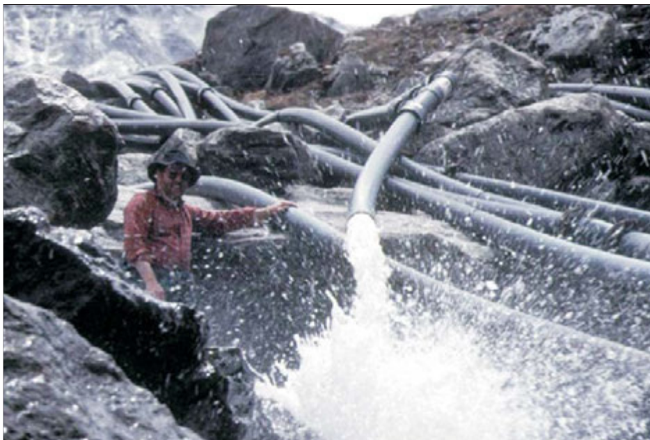
Figure 7.14: Installation of siphons for diverting water from glacial lakes
