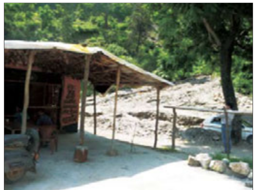
Fig.4.18: Debris flow at Khari poses risk to the shop and school below
