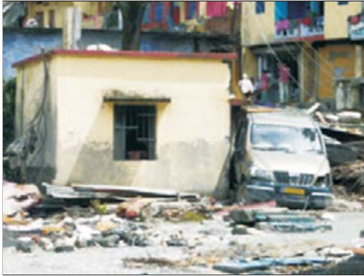
Fig.5.31: Buildings as well as vehicles were destroyed by flashfloods in Asi Ganga River at Gangori
