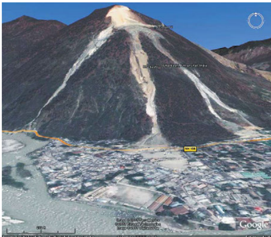
Fig. 2.1: Image of Varunawat Landslide as seen from Google Earth
