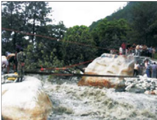
Fig.5.27: Collapsed building situated near Asi Ganga River at Gangori
