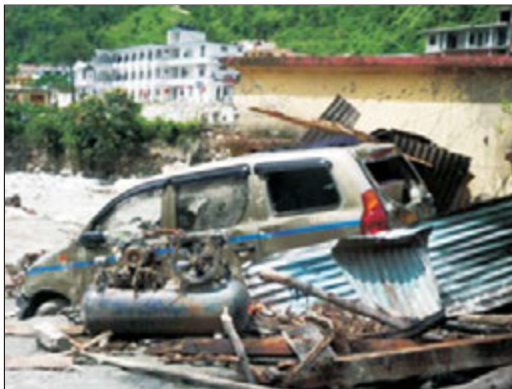
Fig.4.37: Damaged Car and a house after flashfloods in Asi Ganga River at Gangori
