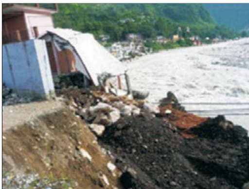
Fig.4.25: Completely collapsed building near Tiloth Bridge at Uttarkashi
