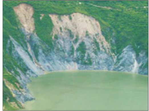
Fig.4.46: Toe induced landslides along reservoir rim of Tehri dam results in land loss and siltation
