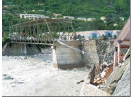
Fig.4.58: A damaged building, connecting road and park near Tiloth bridge after flashfloods
