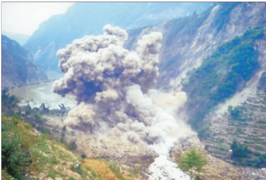
Figure 7.16: Controlled supervised blasting to breach the landslide dammed lake formed after Wenchuan earthquake
