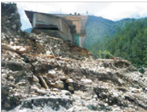
Fig.4.49: A house located on debris slopes lost its foundation partly
