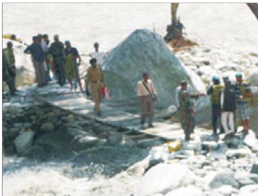
Fig.5.29: A temporary Bailey bridge constructed by BRO after flashfloods in Asi Ganga River at Gangori
