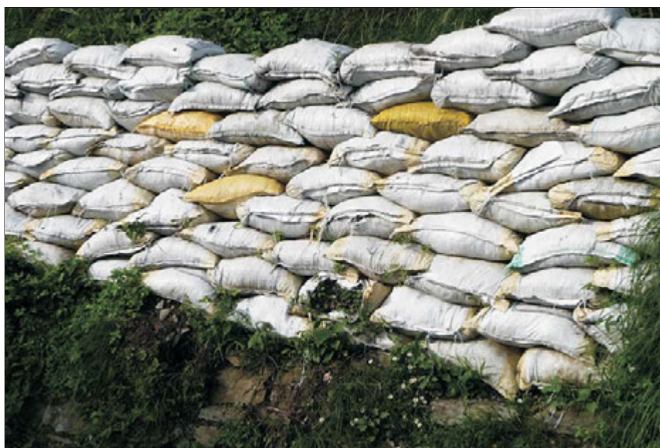
Figure 7.10: Sand-bags used for mitigating the erosion by river water
