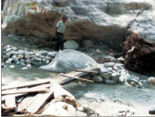
Fig.4.57: A temporary wooden bridge constructed by local community after flashfloods in Asi Ganga River at Gangori
