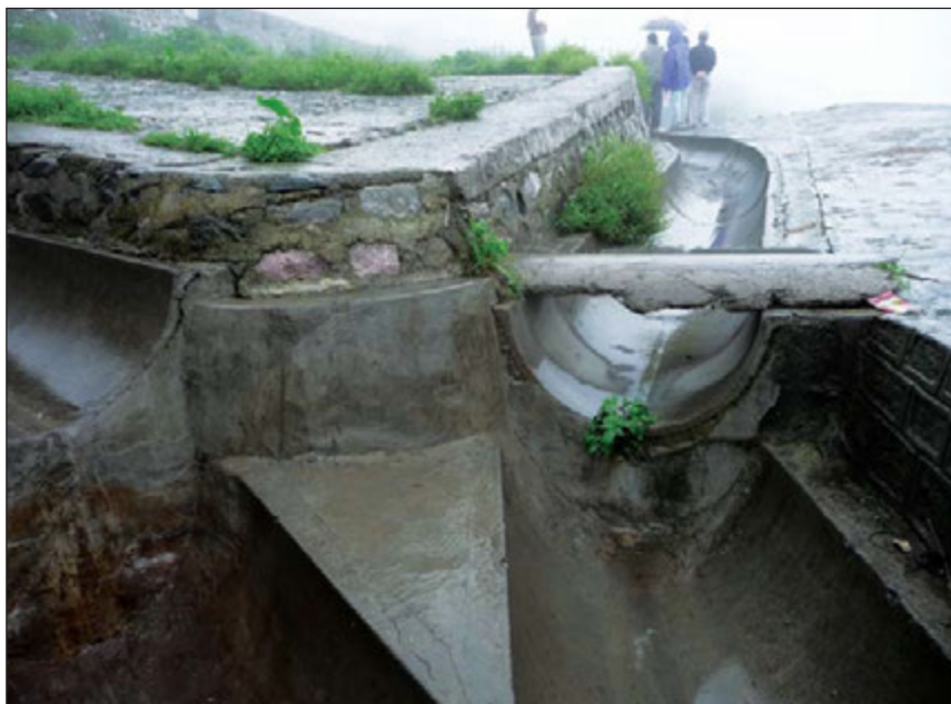
Figure 7.1: Landslide mitigation through lined surface drains
