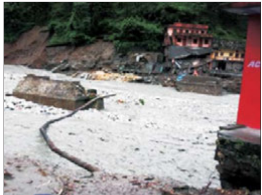
Fig.4.24: River sand and tree logs hit the Ganga Hotel and fill the building
