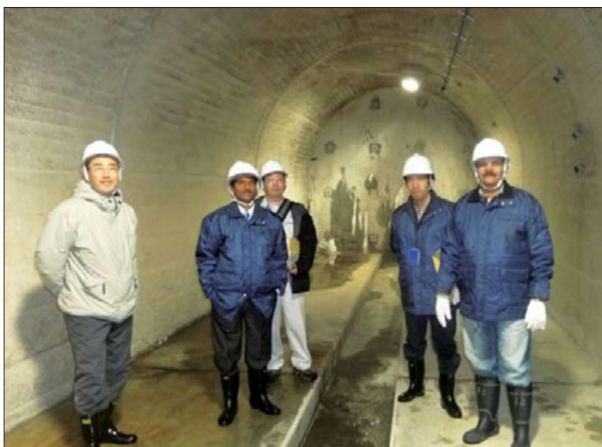
Figure 7.2: Sub-surface drainage works for landslide mitigation
