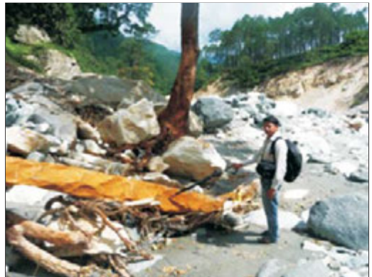
Fig.5.34: Badly damaged water pipeline due to striking boulders during flashflood
