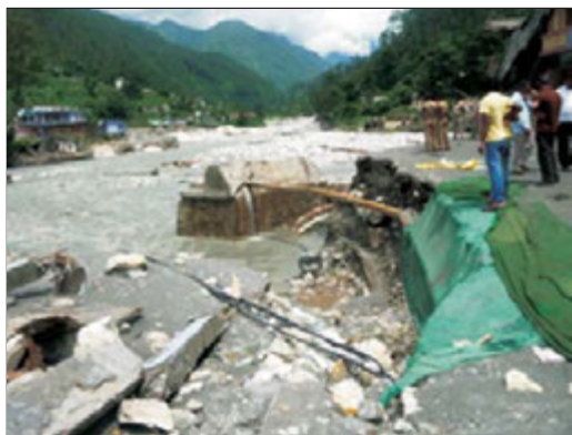
Fig.4.63: Bridge washed away, buildings damaged after flashfloods in Asi Ganga Valley
