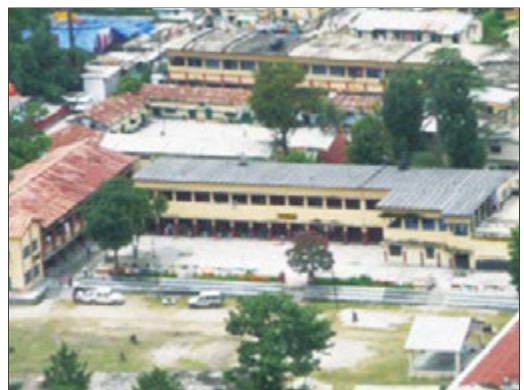
Fig.4.20: Government Inter College where victims got temporary shelter
