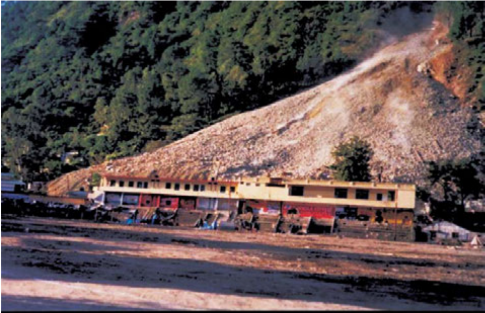
Fig. 2.3: A view after landslide engulfed the hotels shown in the photo Fig. 2.2
