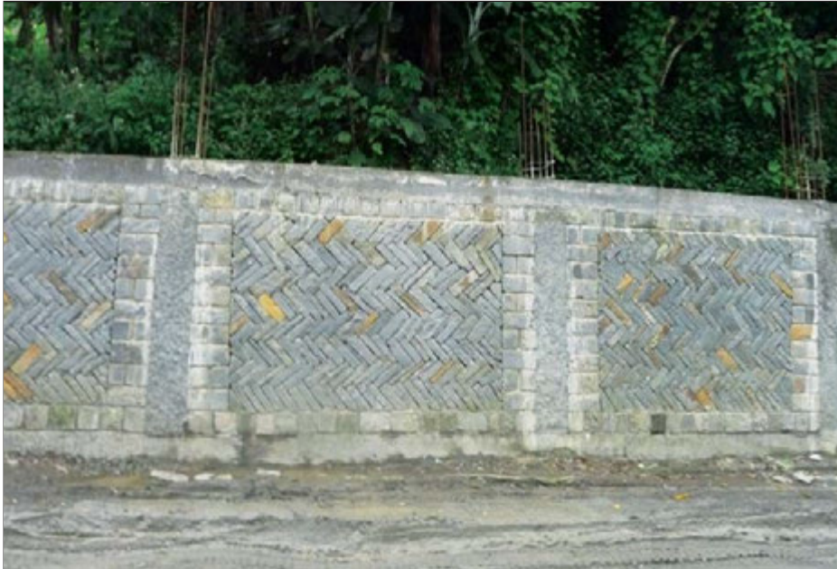
Figure 7.3: Landslide Mitigation using retaining wall made of cut-stones arranged in zig-zag manner bounded with concrete bands
