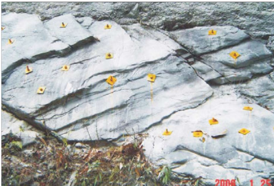
Figure 7.6: Landslide mitigation using pre-tensioned rock bolts
