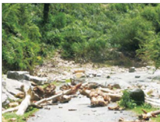
Fig.4.65: Tree logs and boulders seen lying on road after flashfloods in Asi Ganga Valley
