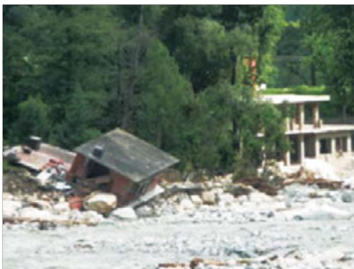
Fig.4.31: Completely collapsed building near Asi Ganga River at Gangori
