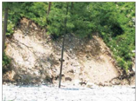
Fig.4.44: Toe induced landslides occurred after flashfloods in Asi Ganga River at Gangori
