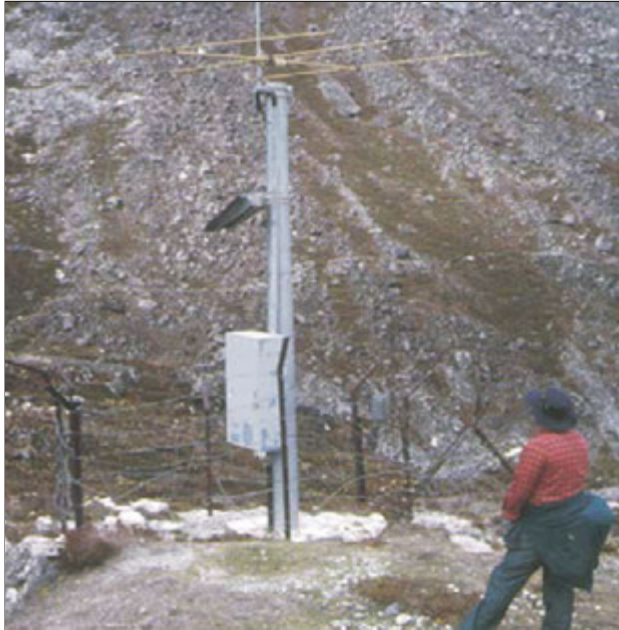
Figure 7.11: Installation of early warning system
