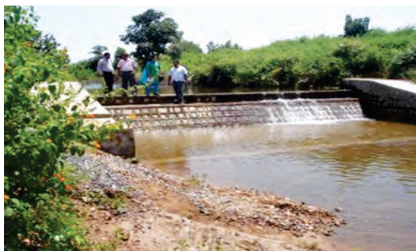
Figure 3.4 Structural Mitigation Measures (Stop dams) in Chopra Village, Datia.
