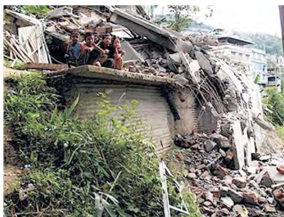
Damaged School building in Sikkim (Photo: Seedsindia)
