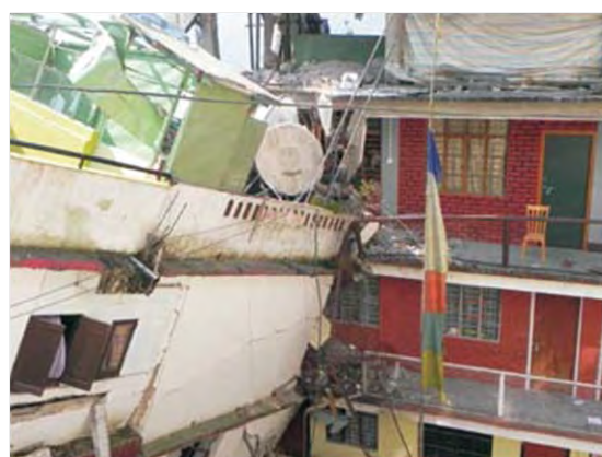
Two buildings at Baluakhani developed excessive tilt on 23rd Sept 2011. Special team from Hyderabad was engaged for demolition. Several buildings in Gangtok have been declared unfit and they are being demolished one by one. However, there is a need to look into the safety of these buildings by experts.
