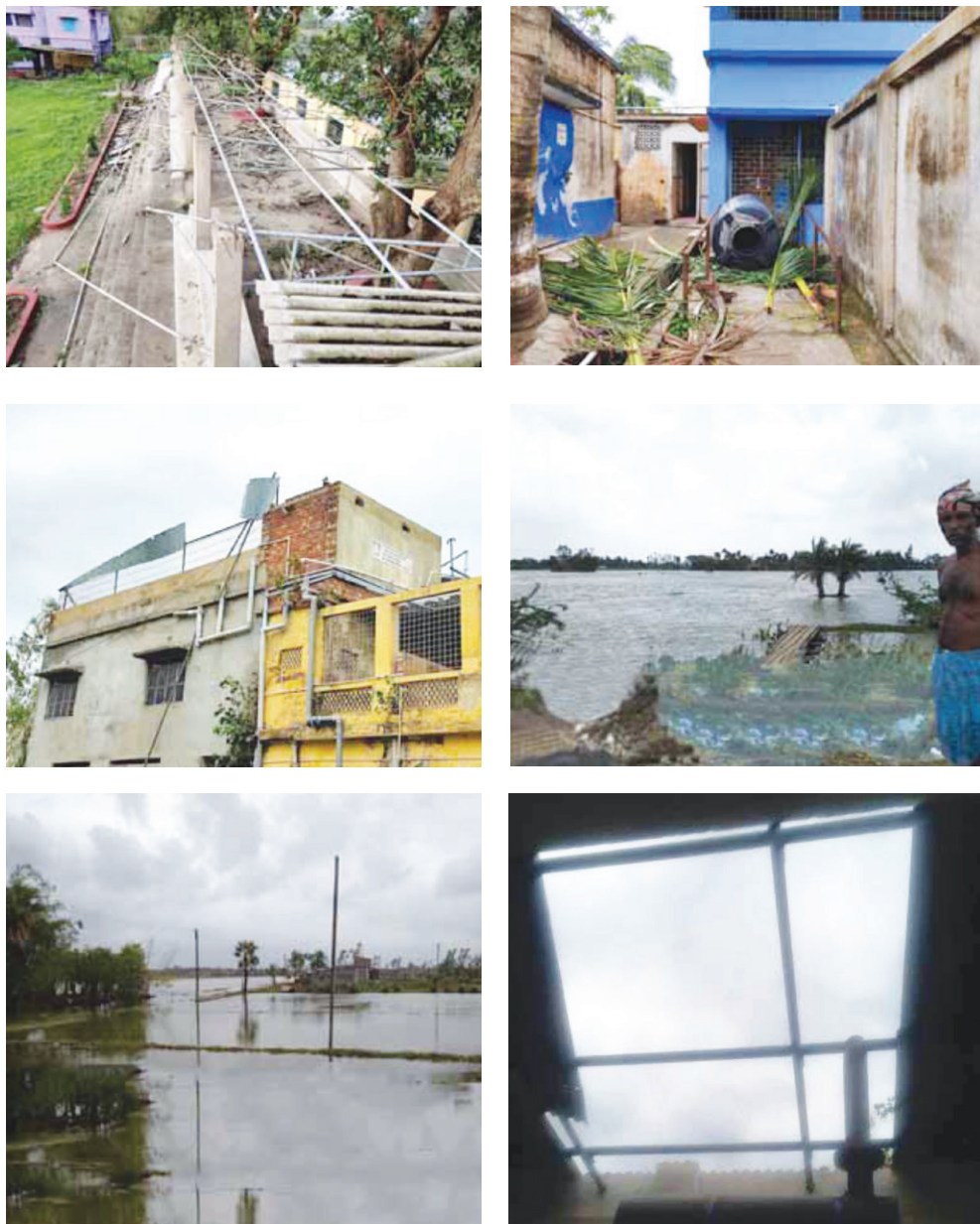
Figure 5.6: Cyclone Yaas - A glimpse of Damages & Destruction in coastal West Bengal. (Source: Government of West Bengal Memorandum on Very Severe Cyclonic Storm, Yaas, May 2021)
