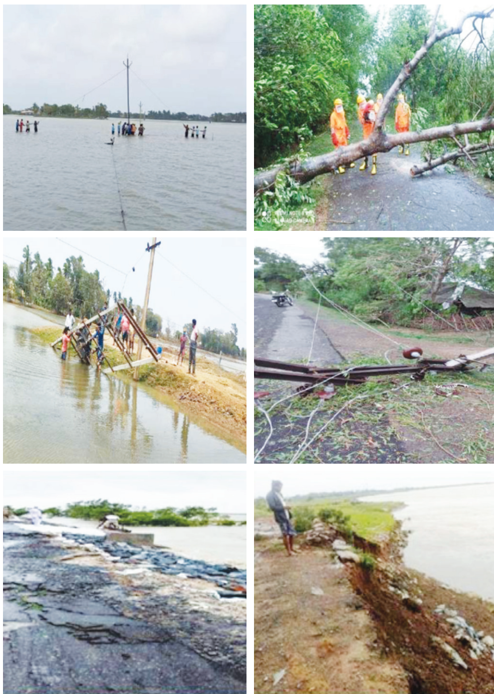
Figure 5.1: Cyclone Yaas - A glimpse of Damages & Destruction in coastal Odisha. (Source: Government of Odisha Memorandum on Very Severe Cyclonic Storm, Yaas, May 2021)
