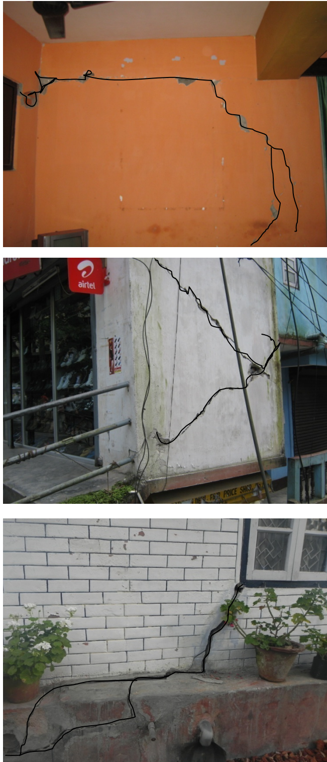
Figure 16 Damages in buildings in and around Gangtok. These cracks are entirely repairable but cannot be assured for enduring moderate shock again
