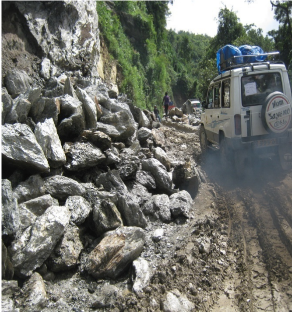
Fig. g-1. Road clearance made upto Mangan, North dist. HQ., in 3 days time after the earthquake but long term performance measures not ensured thus affecting work of power projects,
