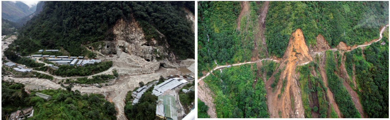
Fig.h. An aerial view of Teesta III hydro power project site partially damaged in Sunday's earthquake in Chungthang, India, Wednesday, Sept. 21, 2011 and aerial view of massive landslides triggered by the earthquake along Gangtok-Mangan highway. (source AP / Altaf Qadri)
