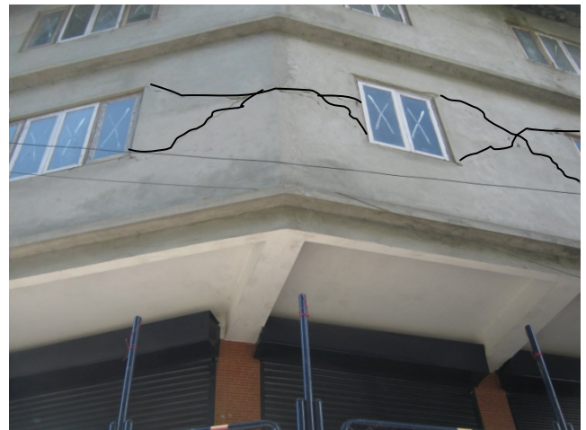
Figure 16 Damages in buildings in and around Gangtok. These cracks are entirely repairable but cannot be assured for enduring moderate shock again
