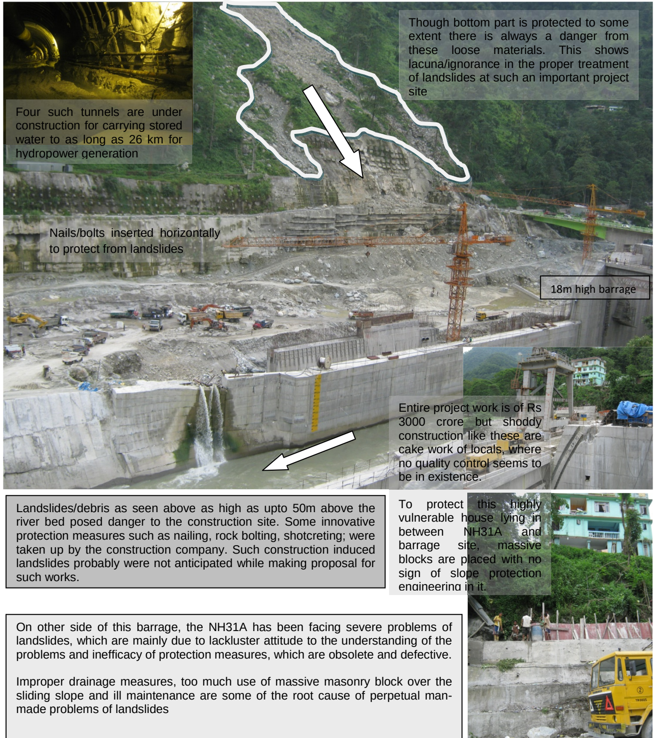
Fig. b. Ongoing Barrage construction site at Sirwani, near Singtam, Sikkim state, along with 26km tunnel for hydropower generation by Lanco Infratech Limited
