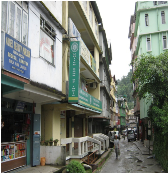
Fig. e-3. Fearing from aftershock effect many residents in Deorali area, Gangtok spend nights in this narrow lane vied with tall buildings. Almost all buildings in this area developed cracks in the partition wall.
