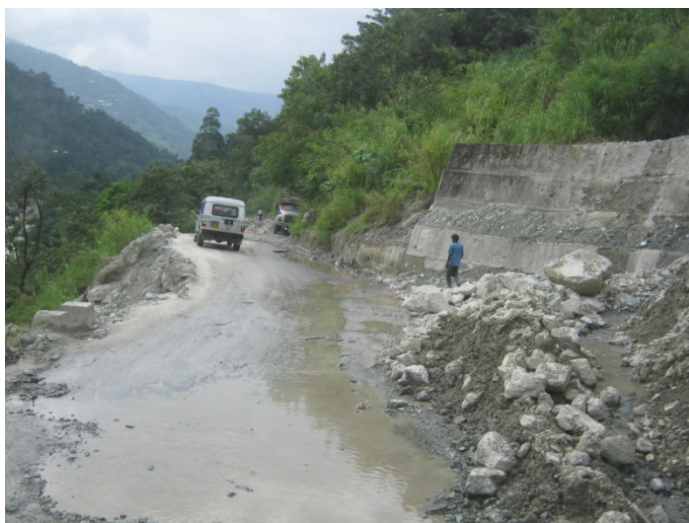
Fig. c-1 Road conditions became worse due to landslides and drains got choked
