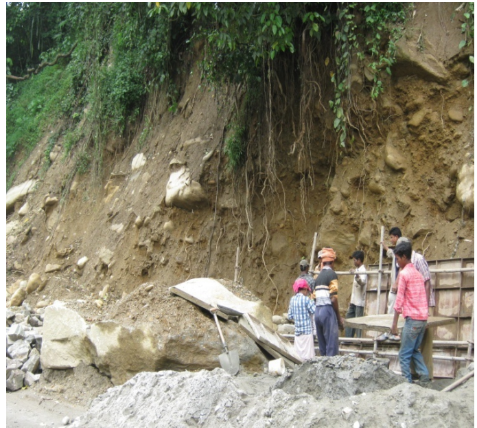
Fig. g-2. Road widening along NH31A near Ranipool is on but technical feasibility of taming cut slope as seen here are very much local and pristine
