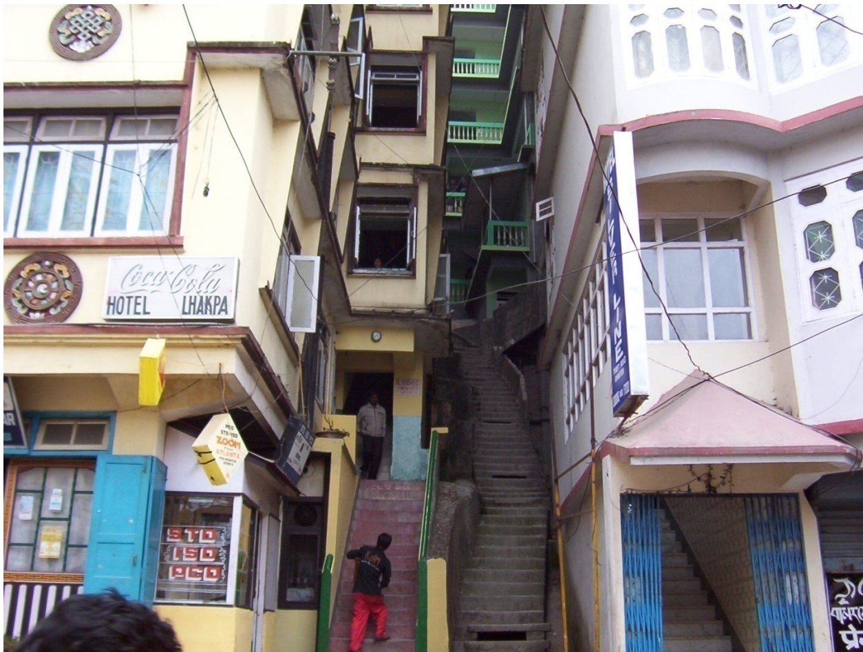
Figure 2 Buildings in Gangtok are standing as high as 8 floors on steep slopes with little or no spaces in between and having all vulnerable components such as floating walls, soft storey, irregular geometry in plan and elevation, etc. Though most of all, as shown above, are having defined load bearing members such as beams and columns, their integrity are subject to performance criteria defined by each visiting earthquake in the region.
