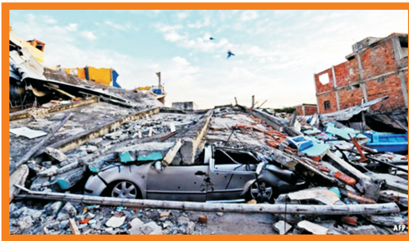
Figure 3. Debris from building collapse after Kumamoto earthquakes in Japan (Source The Economist April 23 2016)
