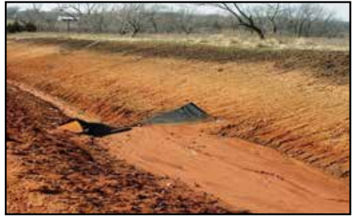
आकृति 3.61: अवरोधक तटबंध (Source: http://www.calpaclab.com/silt-dike-runoff-protection-erosion-control-barrier/ut-9712 )
