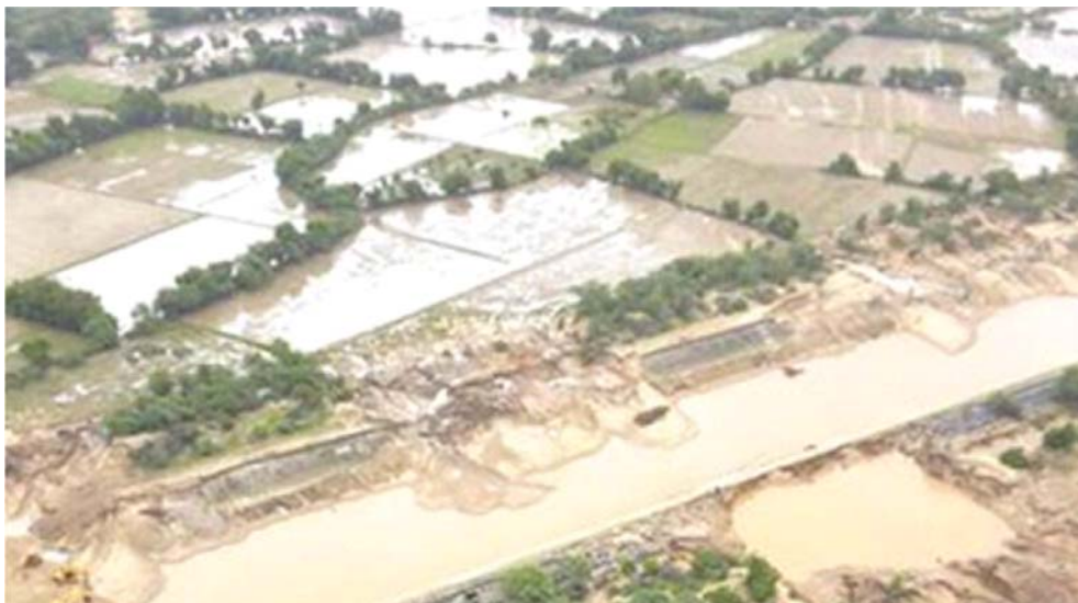
Figure 22: Aerial photograph shows that the canal has been breached at several places. (Source: https://indianexpress.com/article/india/gujarat-floods-the-deluge-4775591/ )
