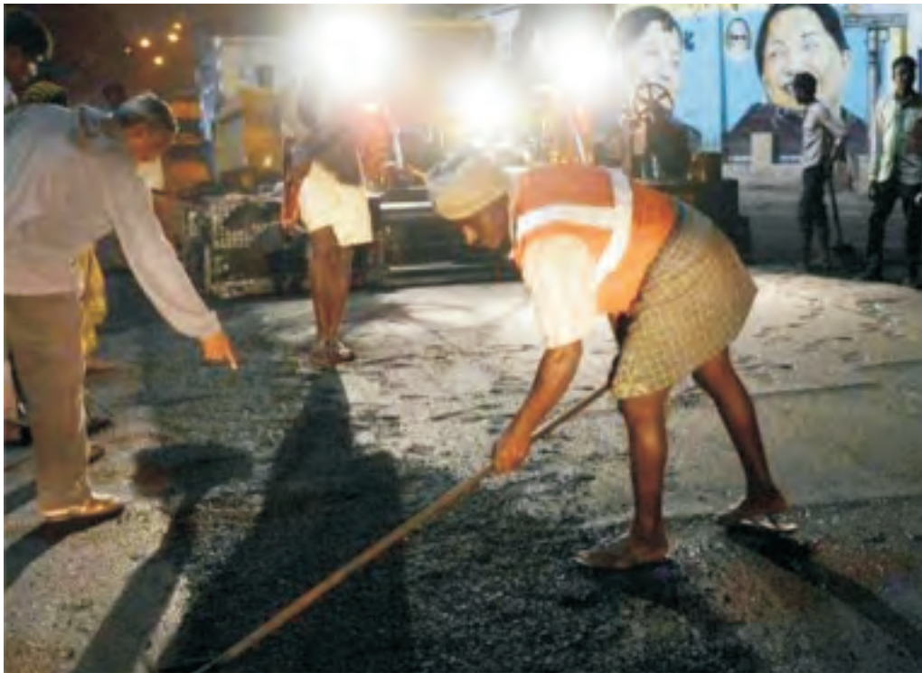
Figure 5.14: Repairing works of Roads by the Civic Authorities Source: The Hindu
