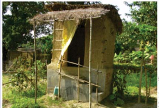
Raised, waterproofed substructures were built with project support (top). Households added their own superstructures (bottom).
