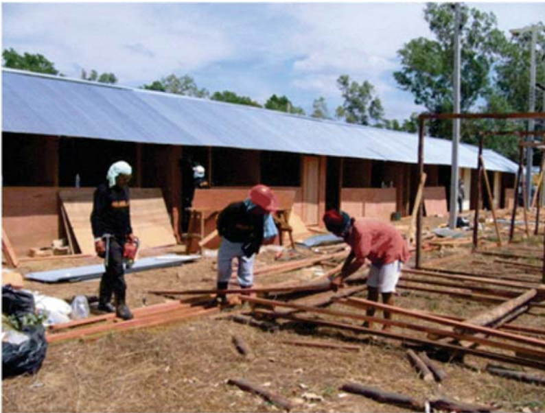
Figure D-2: Post Tsunami Community Members and Volunteers Working for Temporary Housing.
